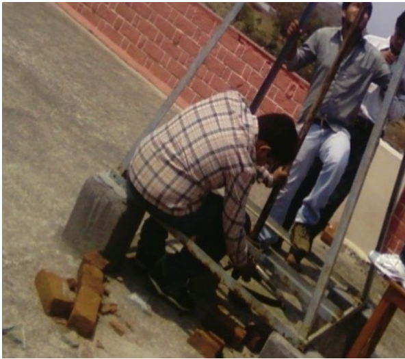
Figure 6: Fitting Stand above Concrete Pillars
